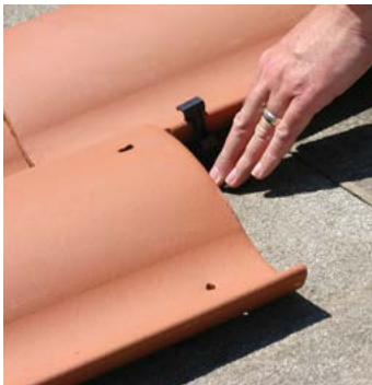
Tall Clip Direct Deck Installations on US Tile® Clay “S” Tile
