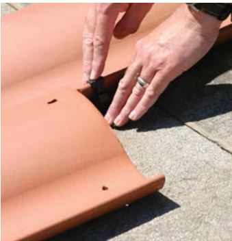
Tall Clip Direct Deck Installations on US Tile® Clay “S” Tile
